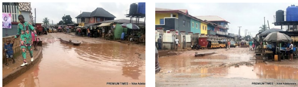
Figure: NDDC road projects in Nomayo community, Ikpoba Okha LGA of Edo state
